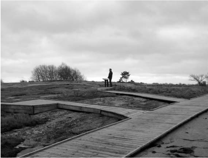
Fig 7. The timber decking under construction. Photo Per Nilsson.
